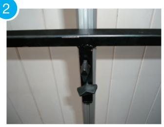
Hold the shelf frame at the required height and tighten the wing nuts to keep the shelf in place.
